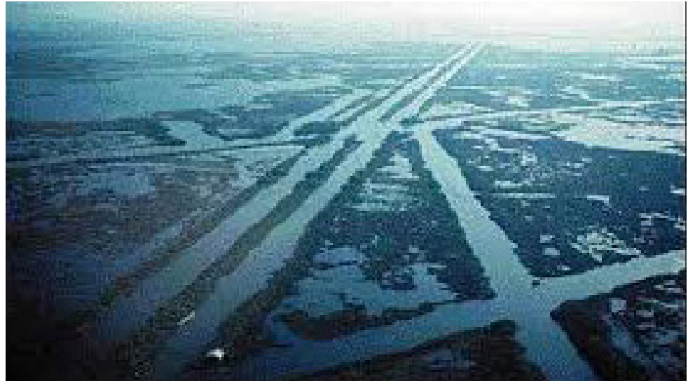
Oil and gas canals through coastal marshes south of New Orleans
